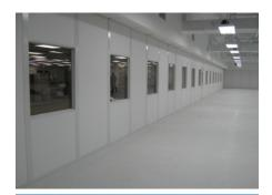
Modular partition walls are easy to assemble and can be moved or modified into new configurations as needs change.
