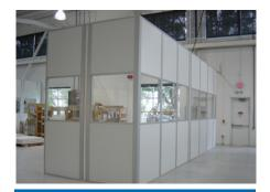
Modular wall panels can be stacked to accomodate extra tall ceilings inside factories like this one. Single span panels are also available to address overheight applications
