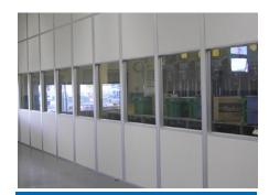
Modular walls offer a functional and attractive alternative to conventional stick and drywall construction. Prefinished panels are easy to assemble and create virtually no mess in the area of construction.
